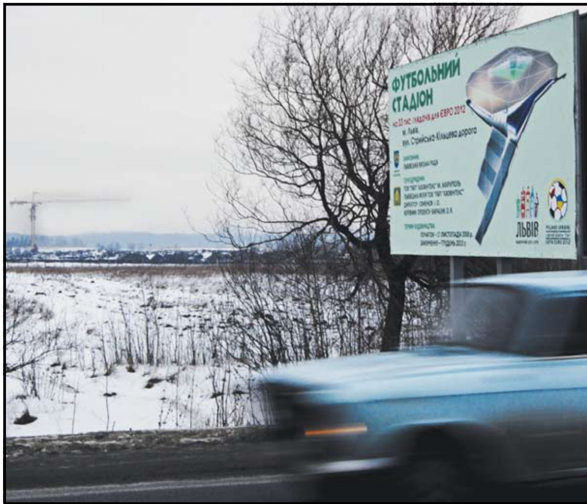
Stadium construction in Ukraine is well underway but the need for new roads is pressing Photograph: AP
